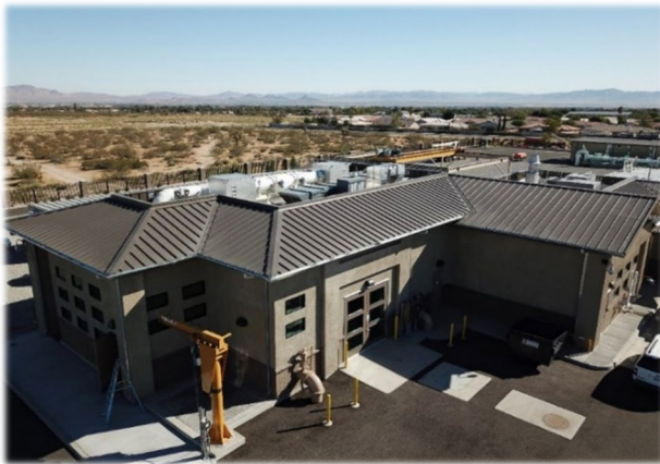
Hesperia Wastewater Reclamation Plant
