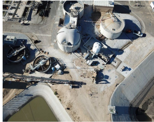
Regional Plant Digesters
