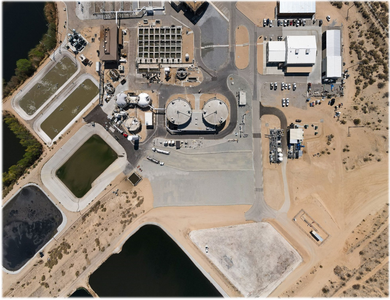
VWRA Regional Plant
