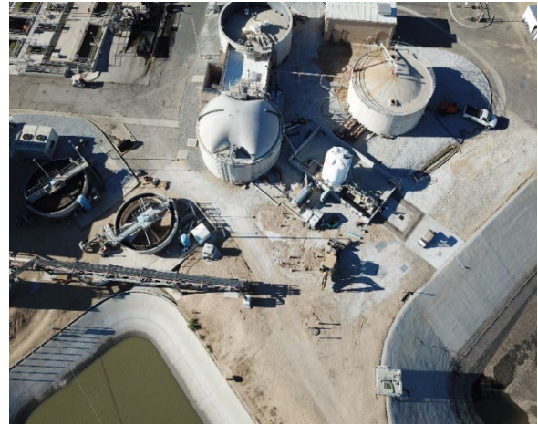
Regional Plant Digesters
