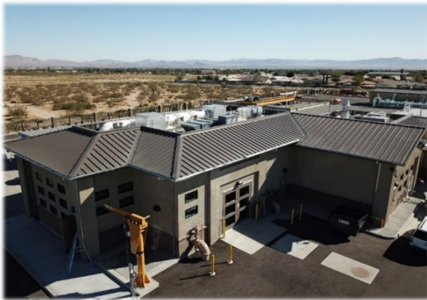
Hesperia Wastewater Reclamation Plant
