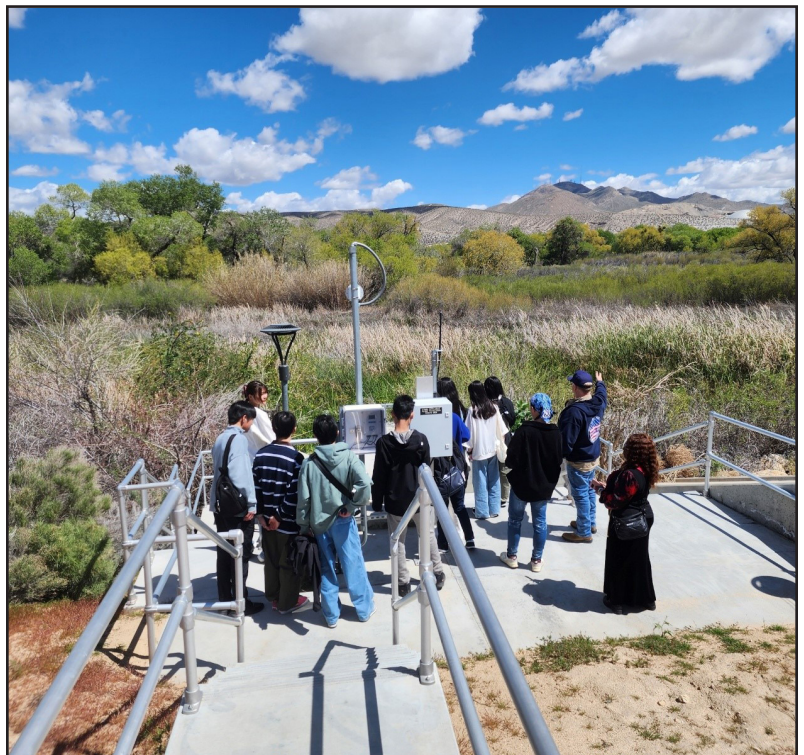
Students get a glimpse of the “outfall” where recycled water from VWVRA is returned to the Mojave River where it replenishes our aquifer.
