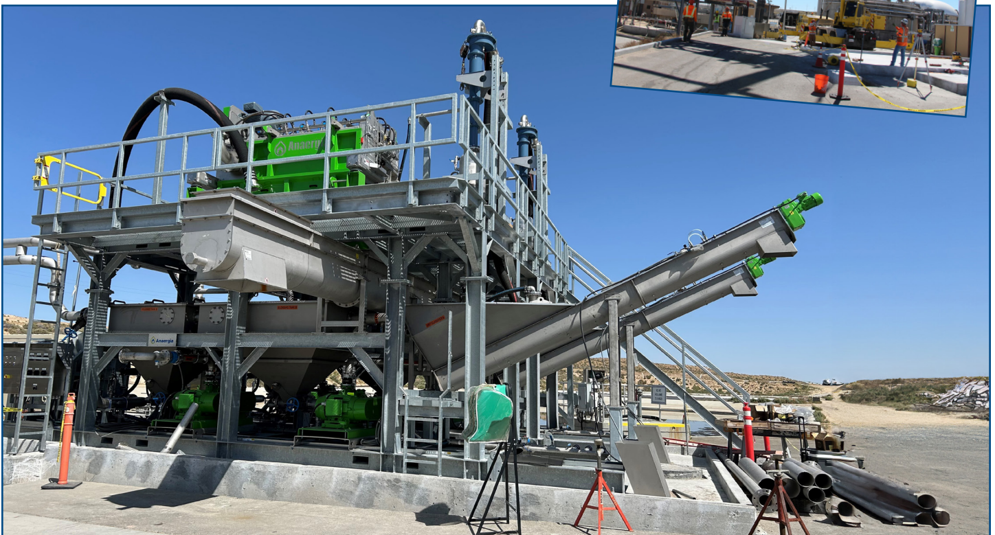
Nearly completed grit removal system.
