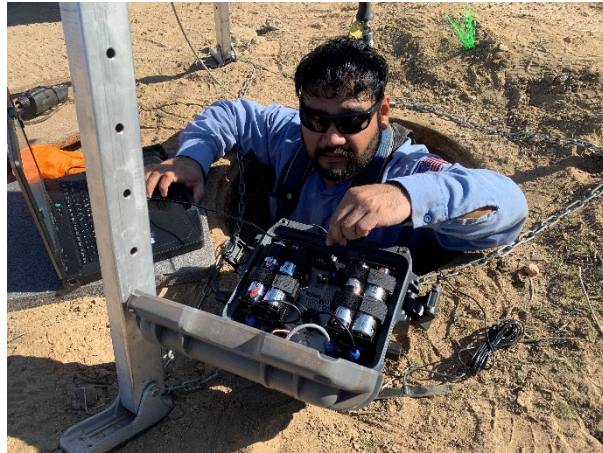
EC Inspector Confined Space Entry
