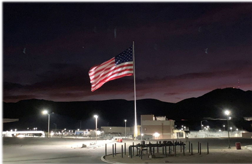
VVWRA Regional Plant Flag
