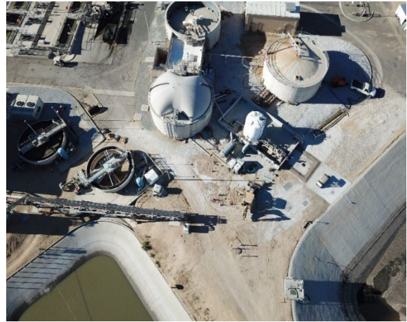
Regional Plant Digesters
