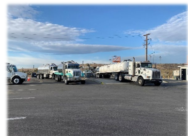
Septage Receiving Station
