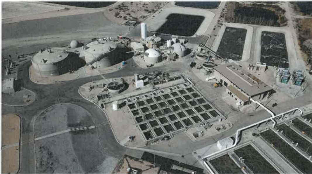
VWRA Regional Plant
