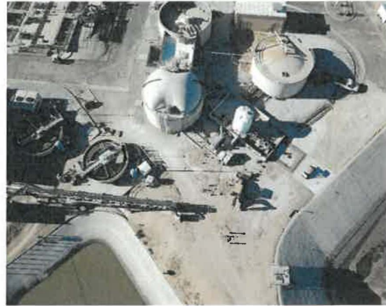
Regional Plant Digesters
