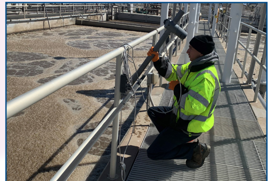
Plant operator Daniel Kessell performs maintenance on probes in the aeration basins.
