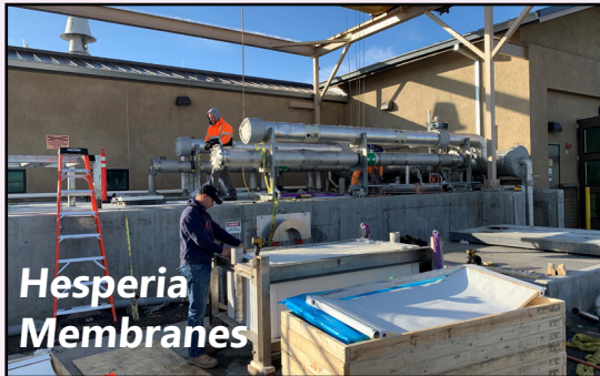
Workers replace the filter membranes at the Hesperia Subregional.
