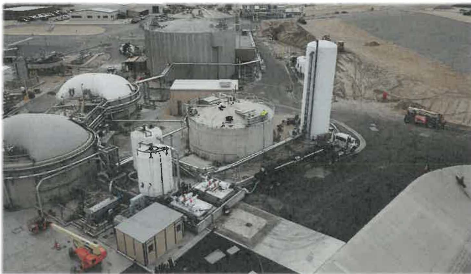
Renewable Natural Gas Project
