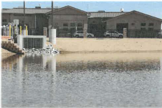
Hesperia Wastewater Reclamation Plant
