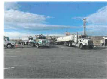
Septage Receiving Station
