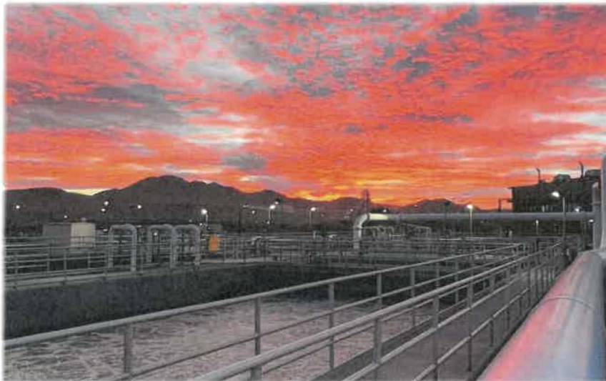
VWRA Regional Plant
