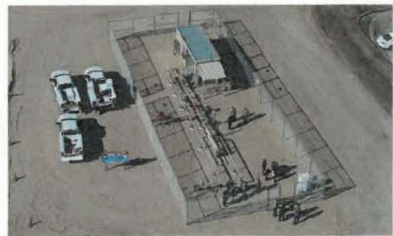
Guests tour the Southwest Gas injection site.
