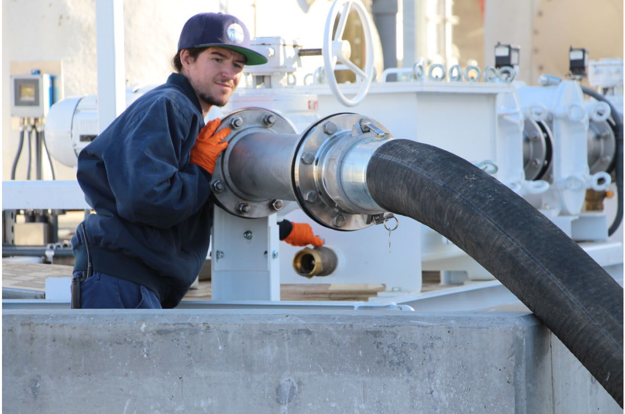
VVWRA's Brandon Talley watches as the first load of food waste is pumped into the digesters.
