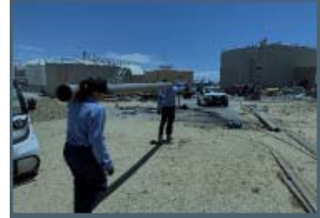
Regional Plant Digesters
