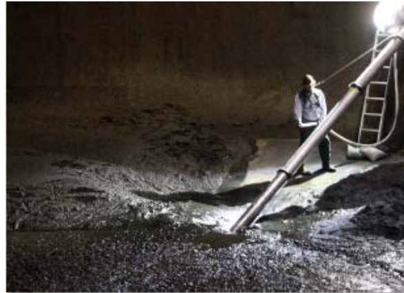
Inside the Digester Building at the Regional Plant
