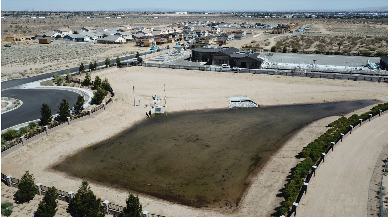
Hesperia Sub-Regional Plant
