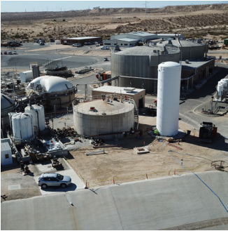
Digesters break down food waste.
