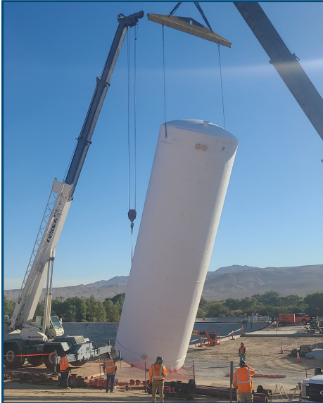
Installation of a 50,000 gallon tank for storage.
