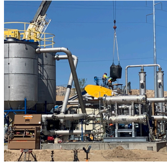
Gas is scrubbed and pressurized to become RNG.
