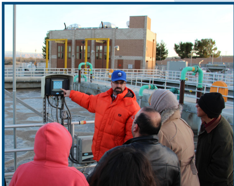
VWVRA GM Logan Olds explains how the monitoring system works for one of our aeration basins.
