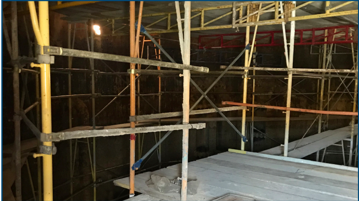
Scaffolding inside digester #3.
