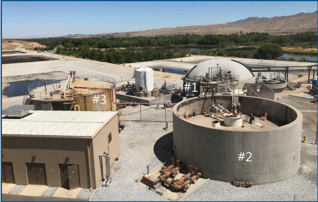
Workers remove debris from the inner wall of digester #2.
