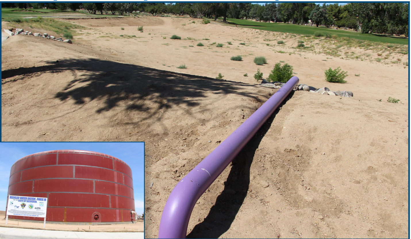
A pond at the Hesperia Golf Course has been plumbed with purple pipe as it awaits delivery of recycled water. Purple pipe is always used to deliver recycled water to any site.
