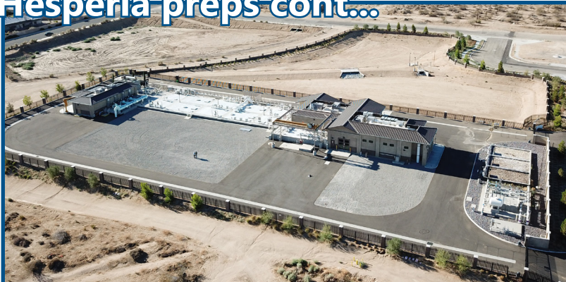
Aerial view of the Hesperia Water Recycling Facility.
