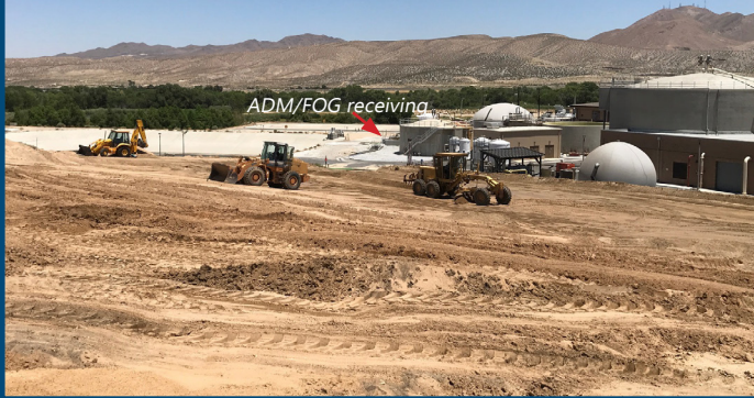
Grading for FOG/ADM receiving road and staging area.
