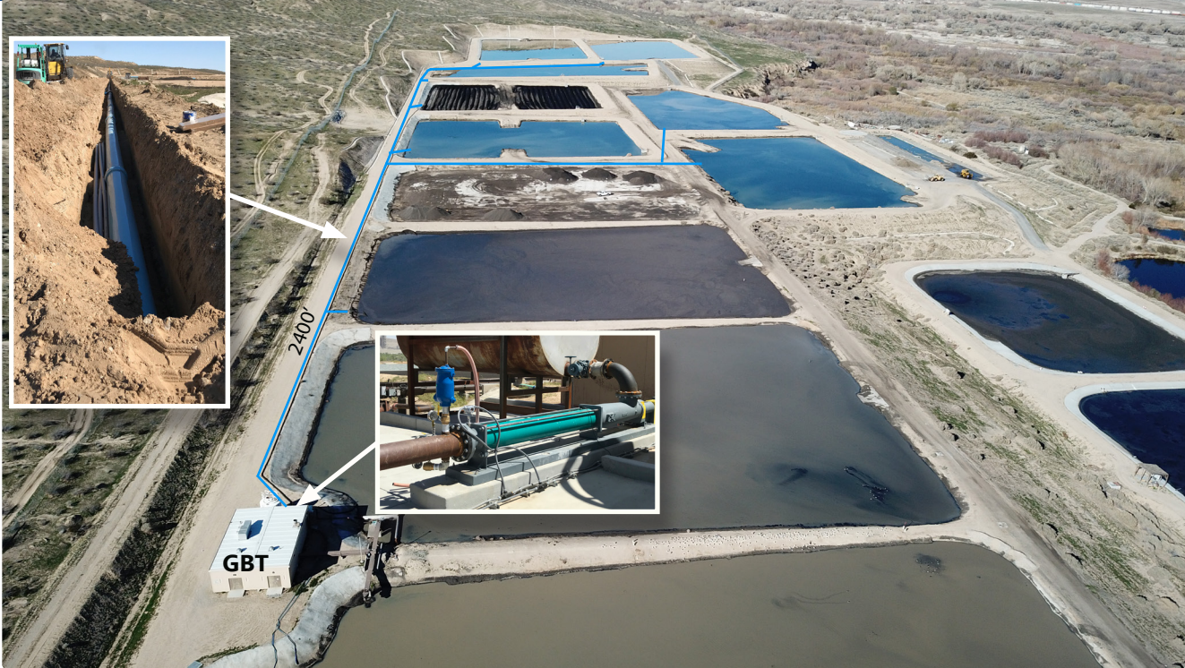
Aerial shot of VVWRA drying beds. Blue line represents the new pipeline installed from the gravity belt thickener (GBT) to the drying beds.
