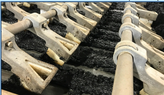
Sludge being dewatered on GBT belt.
