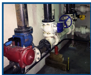
Some of the reconfigured piping in the digester basement.
