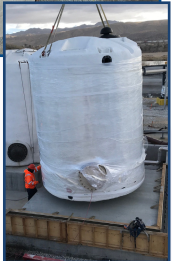
Workers set a new 10,000 gallon ADM tank in place.
