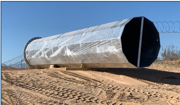
A large base section of power pole waiting to be installed.
