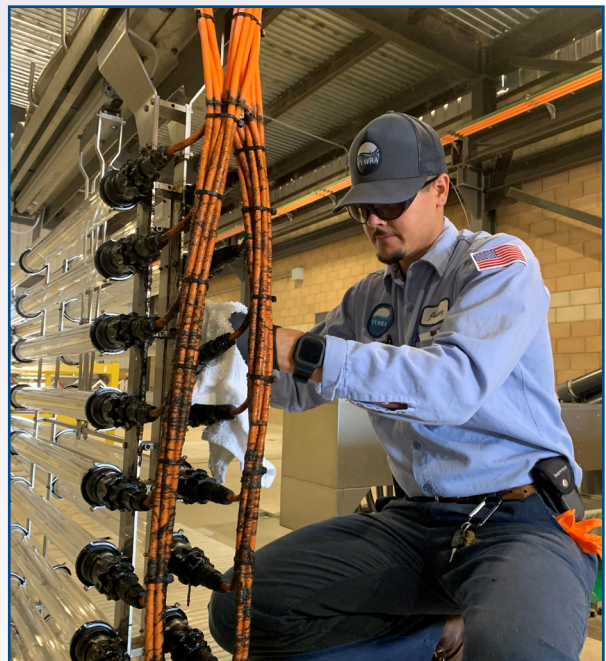
Senior Operator Johnny Bustos prepares to replace UV light bulbs used in the ultra violet light disinfection process. UV light is the final treatment before recycled water is ready to use.
