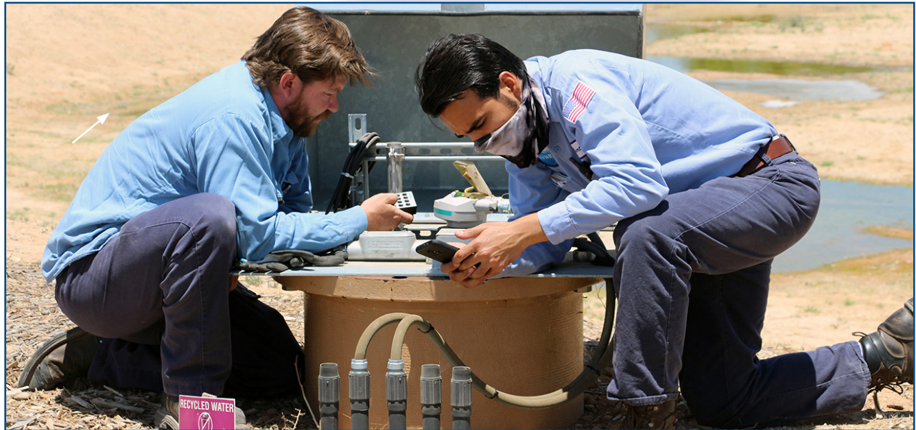
E & I Technician Derek and E & I Intern Adalberto Arteaga perform maintenance on a level indicator and other electronics used to monitor the recycled water percolation ponds at the Apple Valley Golf Course.
