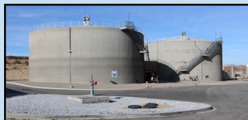
VVWRA's digesters can hold up to 1.3 million gallons of bio-solids each.
