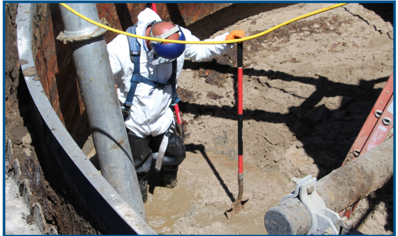
Maintenance mechanic Mike Koncur uses a suction tube from a vacor truck to clean fats, oils, grease and grit from the bottom of a DAFT tank.
