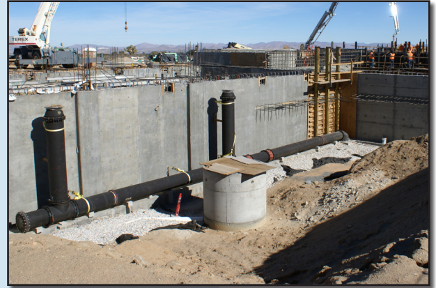
Workers pouring concrete for aeration basins at Hesperia subregional.
