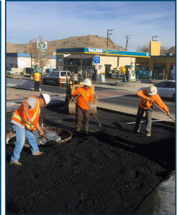
Street being paved with asphalt.
