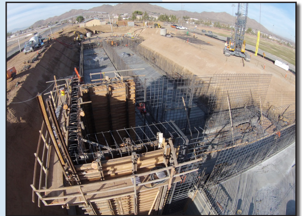
Aerial view of construction of Apple Valley subregional
