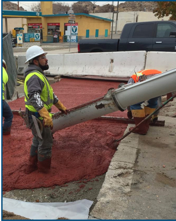
Colored concrete poured.
