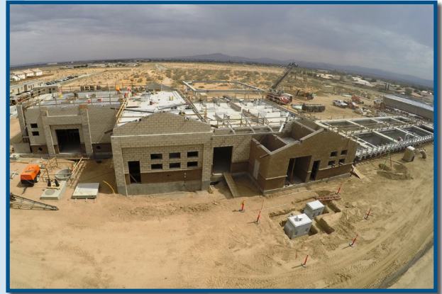
Hesperia subregional construction site.
