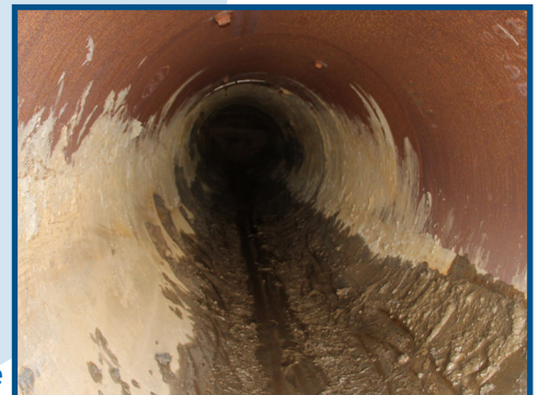
Inside 60" steel casing with mud on the floor.
