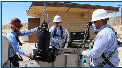
Senior Operator Brad Adams (l), Mechanic Brian Fenton (c) and Mechanic in Training Brad Doneff (r) pull a pump for inspection and cleaning.
