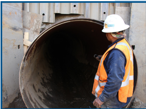
A worker inspects the outside of steel casing.
