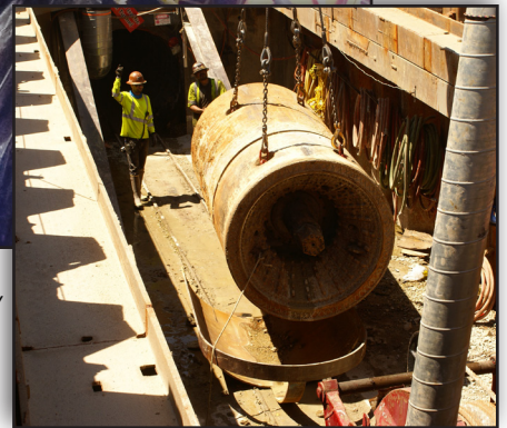
A 12 ton microtunneling machine being pulled from the Upper Narrows tunnel.
