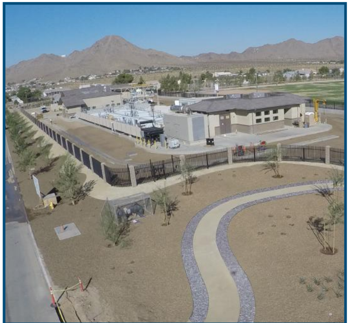
Apple Valley Water Recycling facility looking east to west.
