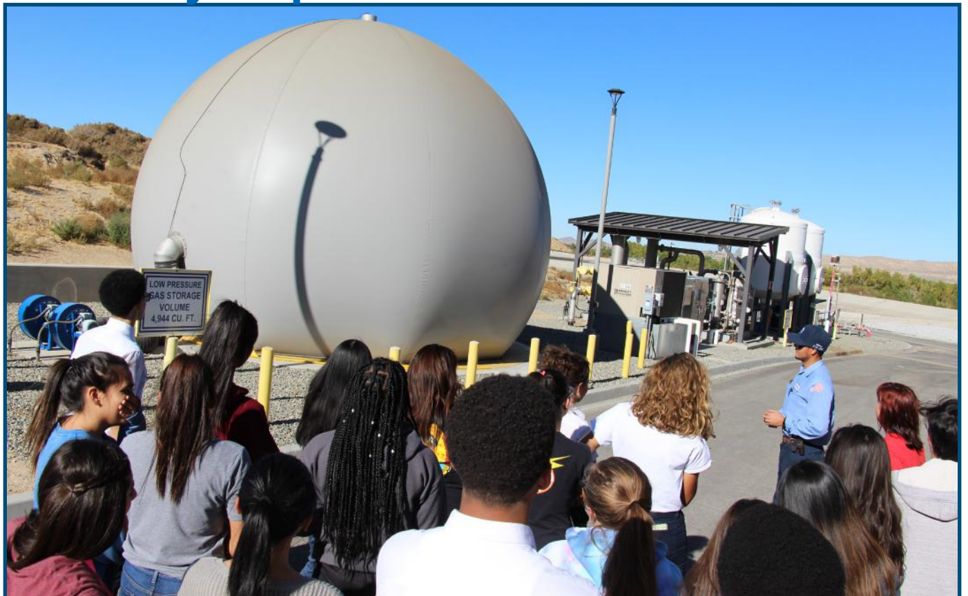
30 science students from University Prep in Victorville recently toured VVWRA's main plant. The tour, led by Sr. Operator Johnny Bustos, included a stop at our large biogas storage bubble. The biogas (methane) collected in the bubble is cleaned and then used to power a pair of 800 kwh generators that produce electricity to power our plant. For tour info, email David at dwyllie@vwwra.com .
