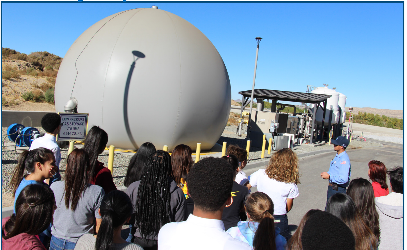
30 science students from University Prep in Victorville recently toured VVWRA's main plant. The tour, led by Sr. Operator Johnny Bustos, included a stop at our large biogas storage bubble. The biogas (methane) collected in the bubble is cleaned and then used to power a pair of 800 kwh generators that produce electricity to power our plant. For tour info, email David at dwyllie@vwwra.com .
