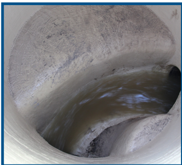
Wastewater flowing through new Upper Narrows pipeline.
