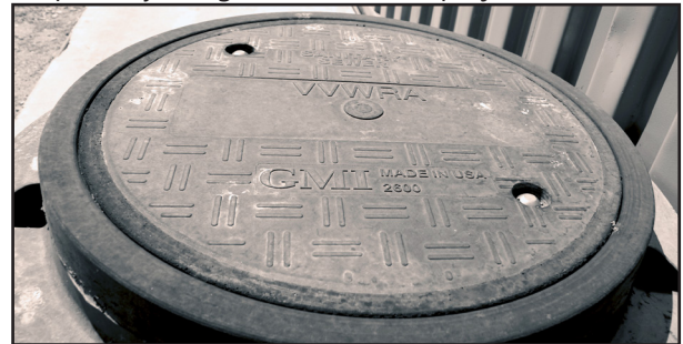
New GMI composite manhole cover
