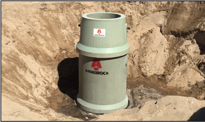
New polymer Armorock manhole installed near Interstate 15 and E St.
