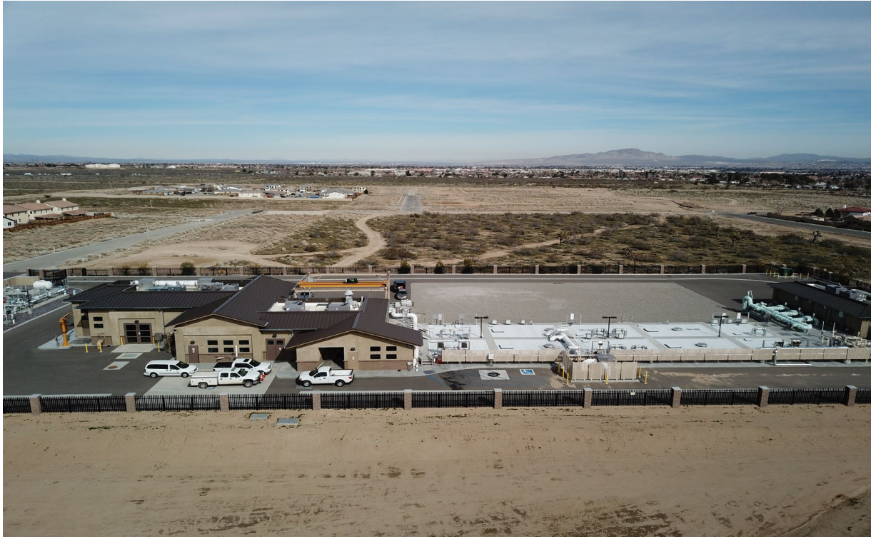
Apple Valley Sub-Regional Water Reclamation Plant
