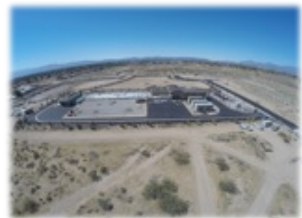
Hesperia Sub-regional Plant
