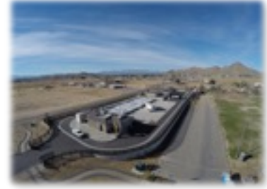
Apple Valley Sub-regional Plant
