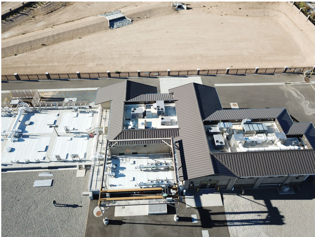
Hesperia Sub-Regional Water Reclamation Plant
