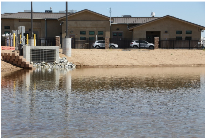
Hesperia Wastewater Reclamation Plant
