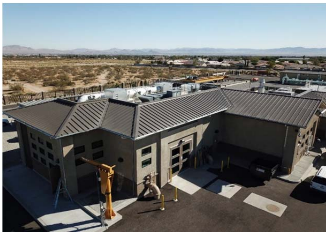
Hesperia Wastewater Reclamation Plant
