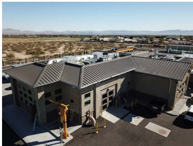
Hesperia Wastewater Reclamation Plant
