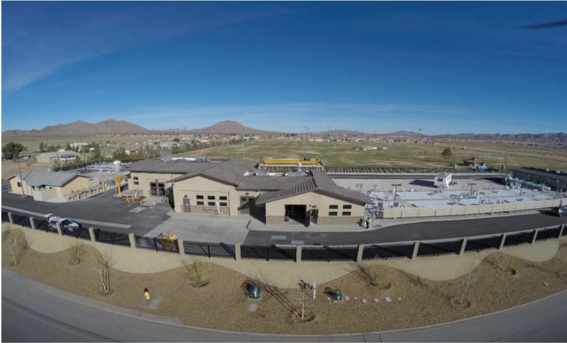
Apple Valley Wastewater Reclamation Plant
