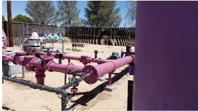
Recycled Water Pipelines
