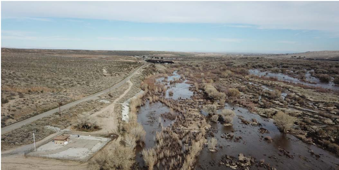
Oro Grande Pump Station
