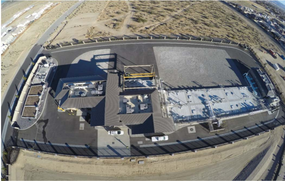
Hesperia Wastewater Reclamation Plant
