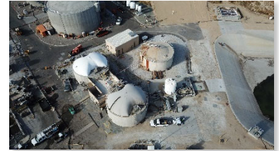
Regional Plant Digesters
