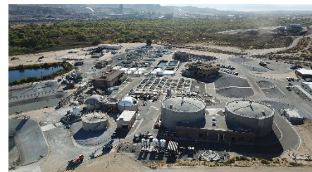
Victorville Regional Plant
