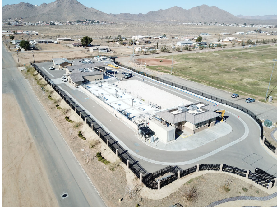
Apple Valley Sub-Regional Water Reclamation Plant
