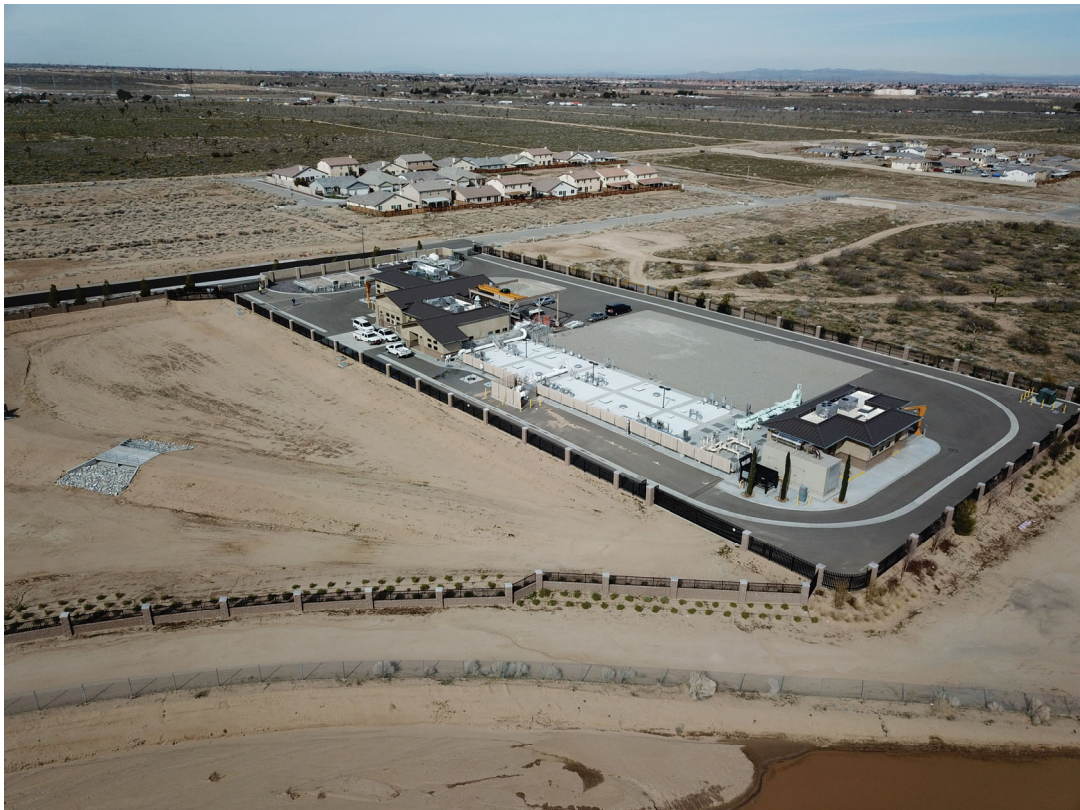
Hesperia Sub-Regional Water Reclamation Plant
