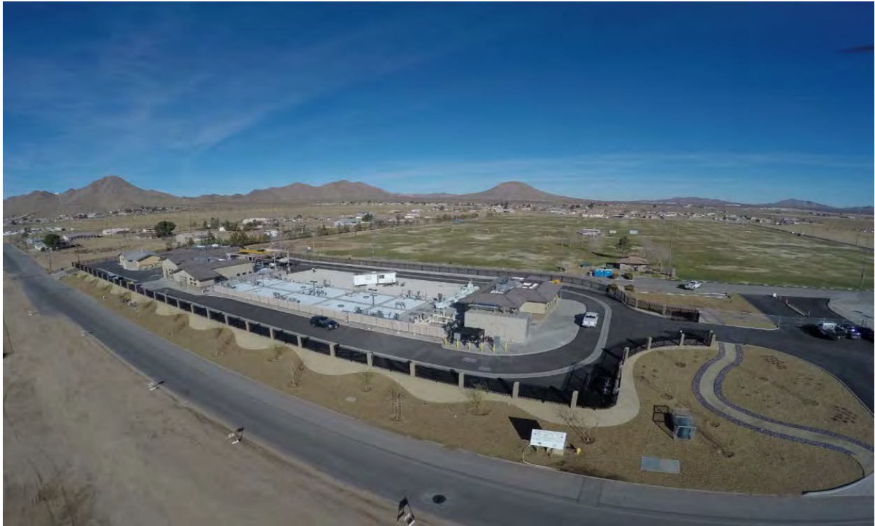
Apple Valley Sub-Regional Water Reclamation Plant
