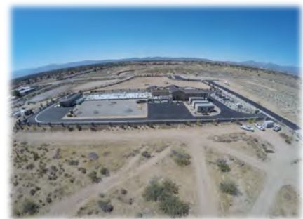
Hesperia Sub-regional Plant
