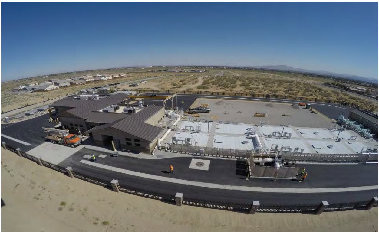
Hesperia Sub-Regional Water Reclamation Plant
