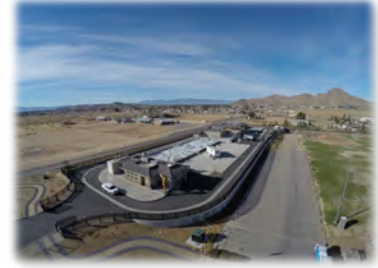
Apple Valley Sub-regional Plant
