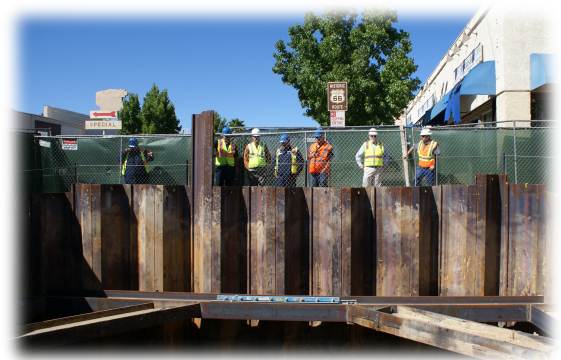
Upper Narrows permanent interceptor construction in progress
