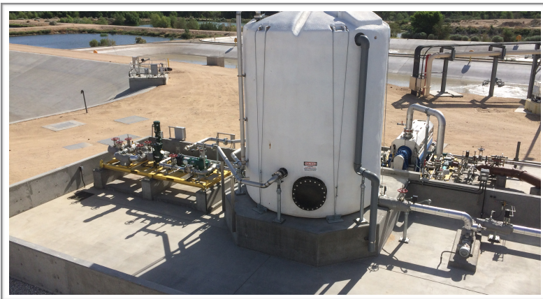
The Omnivore project is underway.
