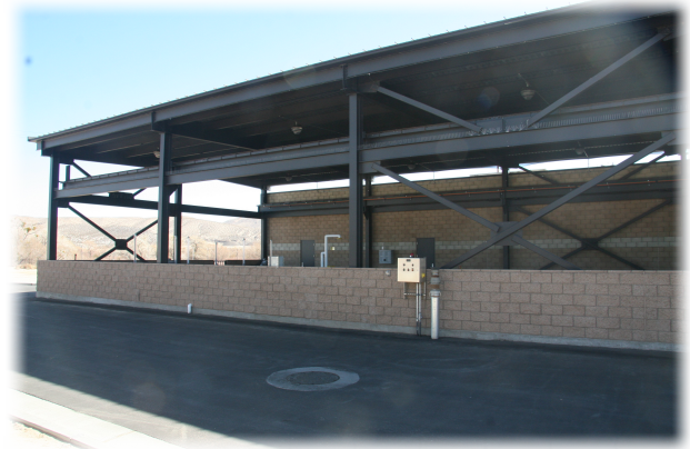
UV System Phase III A Upgrade
