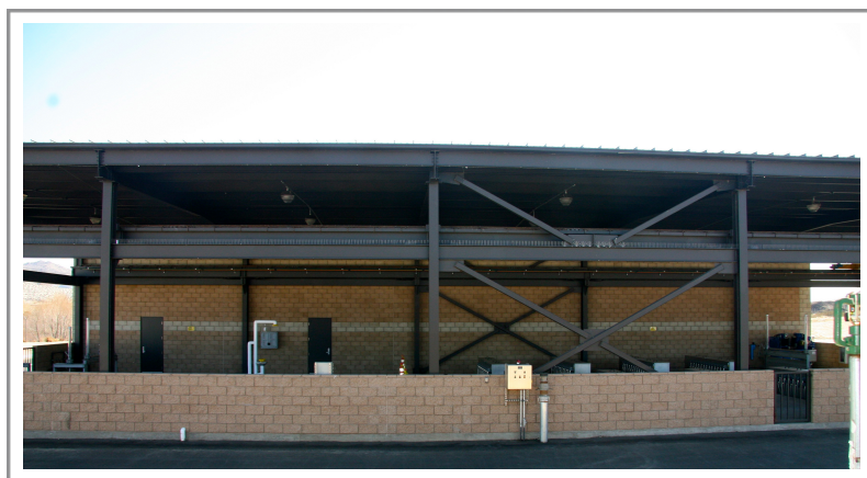
The Phase III A UV System has been completed in August 2013.
