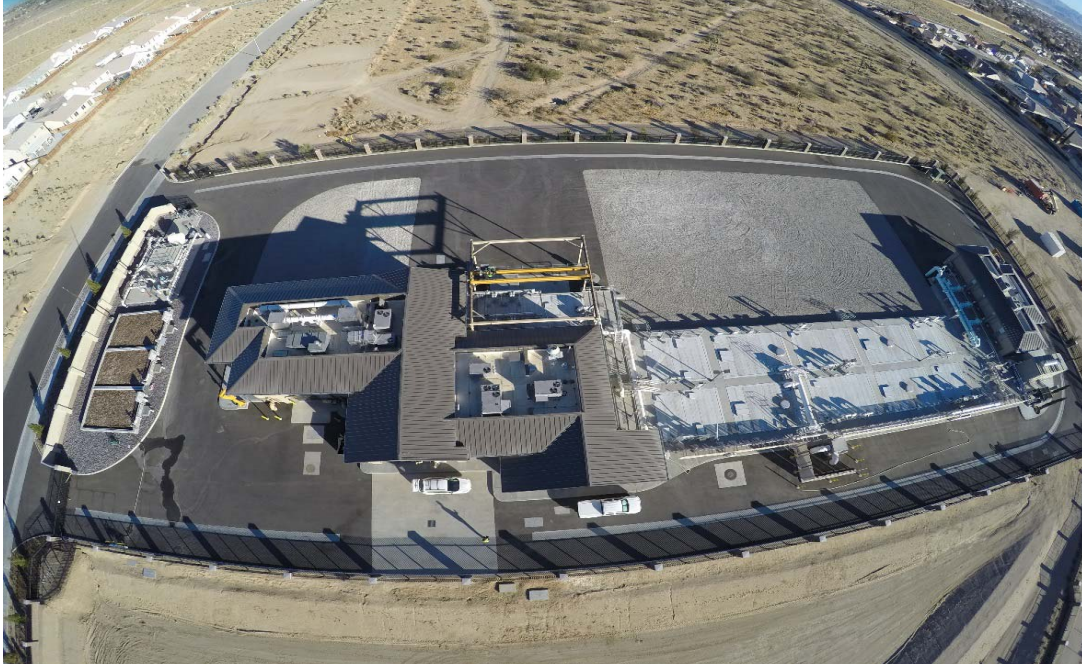
Hesperia Wastewater Reclamation Plant
