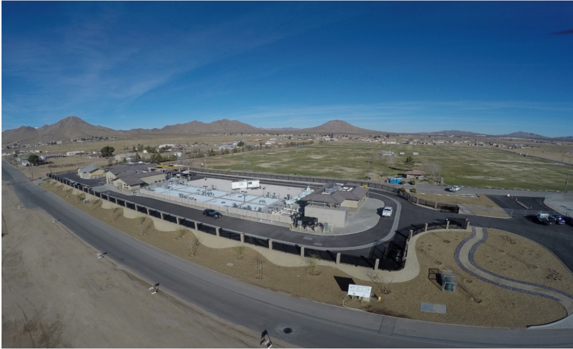
Apple Valley Sub-regional Water Reclamation Plant
