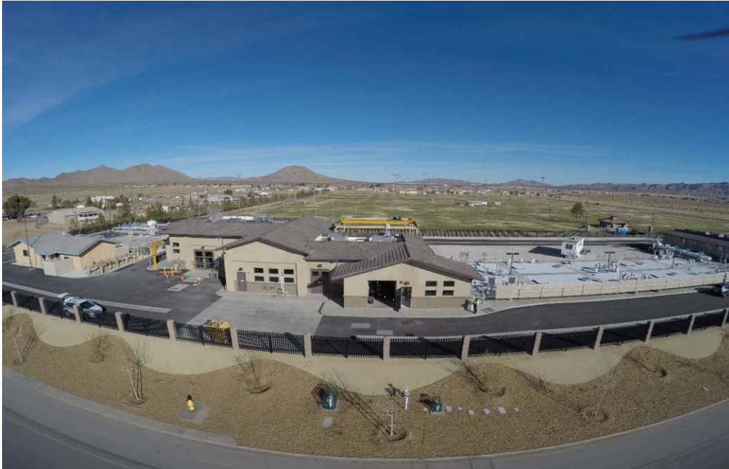
Apple Valley Wastewater Reclamation Plant
