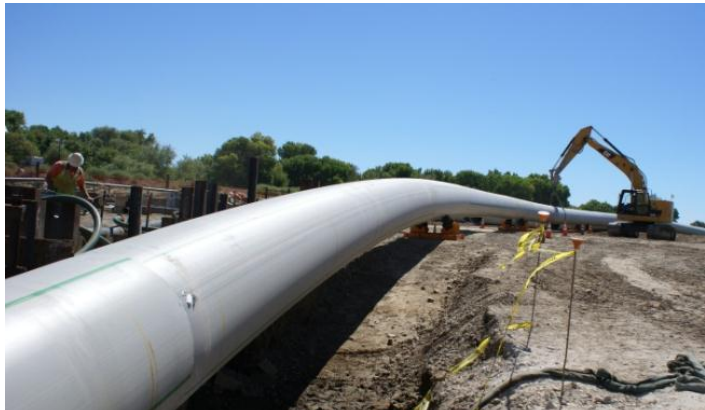
Pipeline for the Upper Narrows Tunnel
