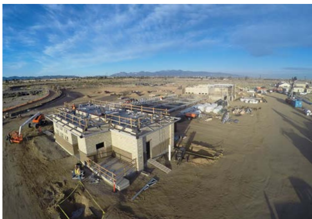
HWRP construction in progress
