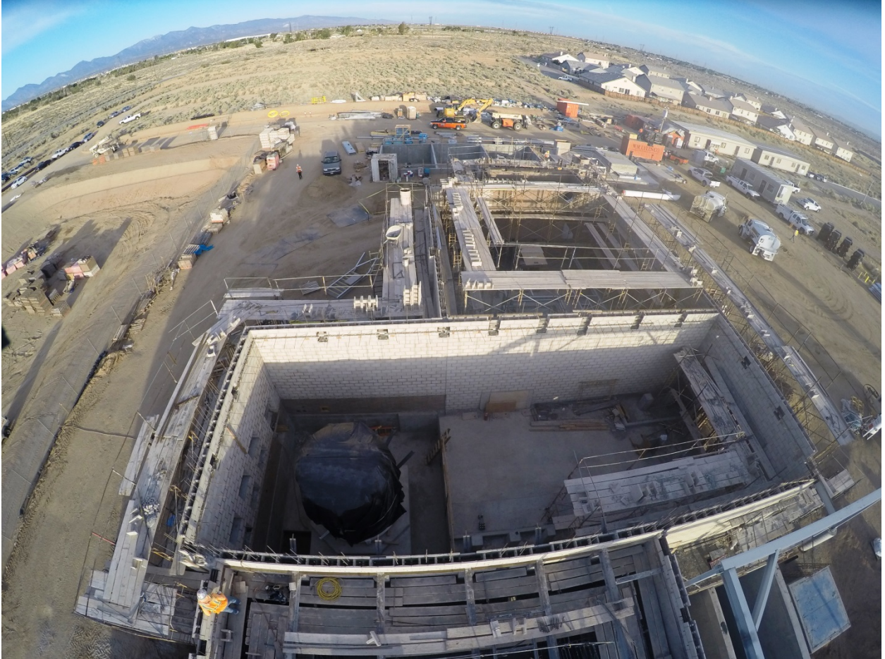
Hesperia Subregional Water Reclamation Plant Project
