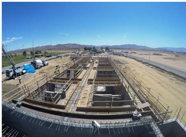
AVWRP construction in progress
