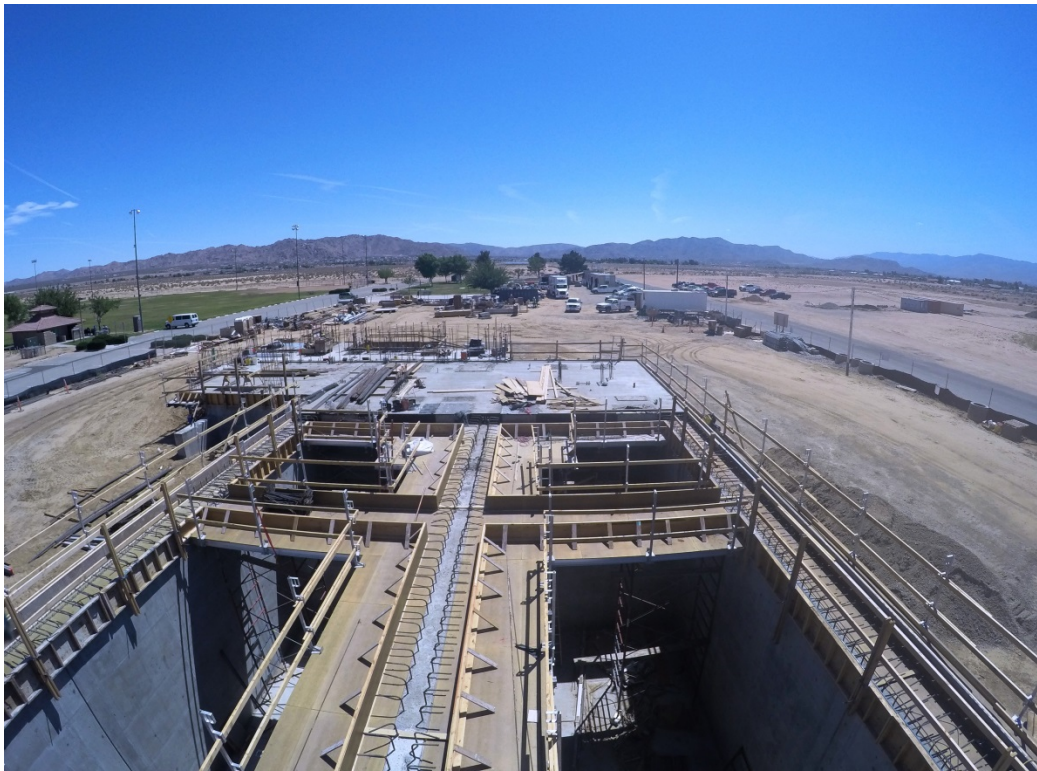
Apple Valley Sub-regional Water Reclamation Plant Project
