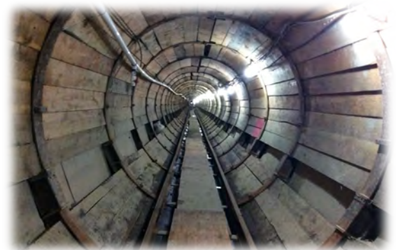
Upper Narrows replacement interceptor construction in progress
