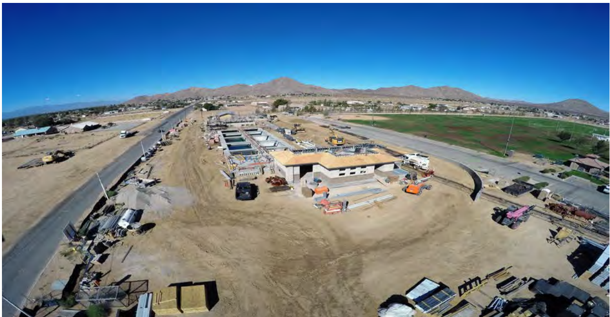
Apple Valley Sub-Regional Plant
