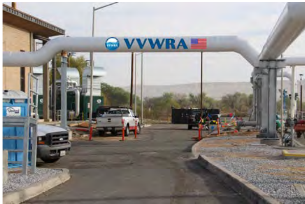
Blower pipeline installation completed
