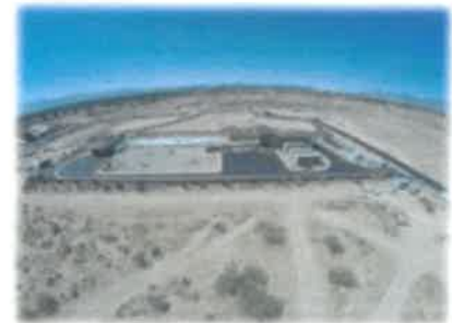
Hesperia Sub-regional Plant
