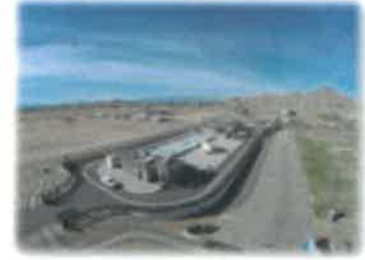
Apple Valley Sub-regional Plant
