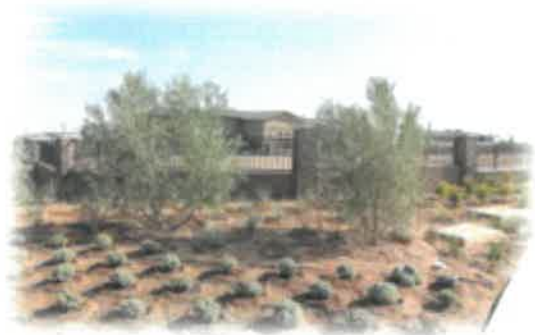
Hesperia Sub-regional Plant
