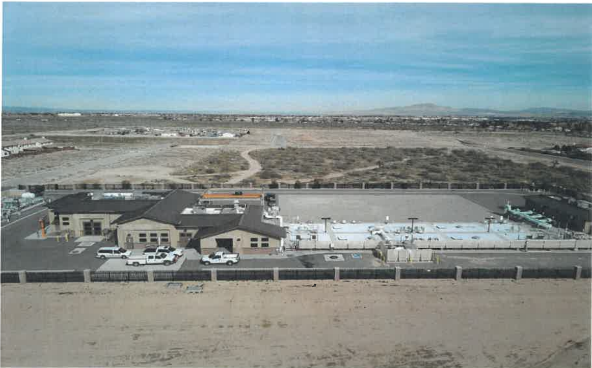
Apple Valley Sub-Regional Water Reclamation Plant
