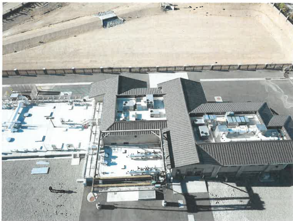
Hesperia Sub-Regional Water Reclamation Plant
