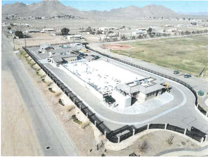
Apple Valley Sub-Regional Water Reclamation Plant
