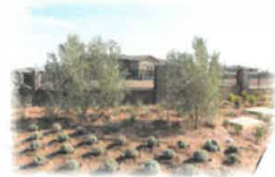
Hesperia Sub-regional Plant
