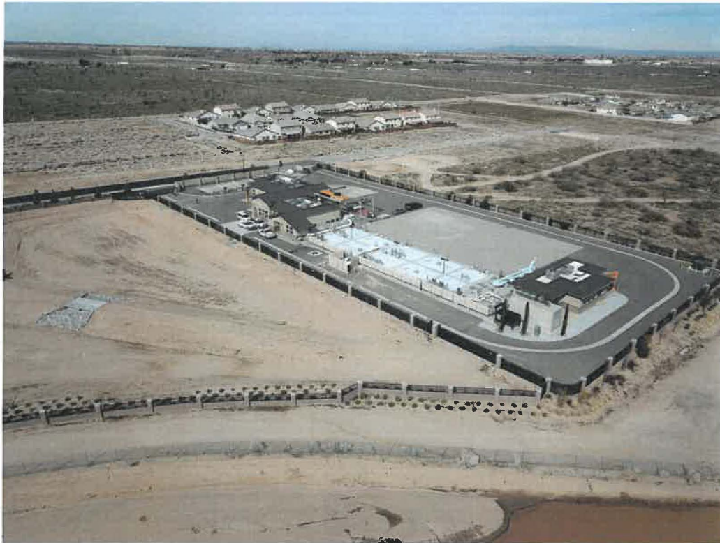
Hesperia Sub-Regional Water Reclamation Plant
