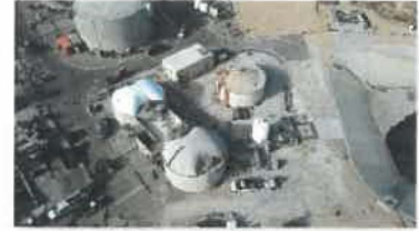
Regional Plant Digesters
