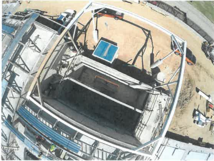
Apple Valley Plant - construction in progress
