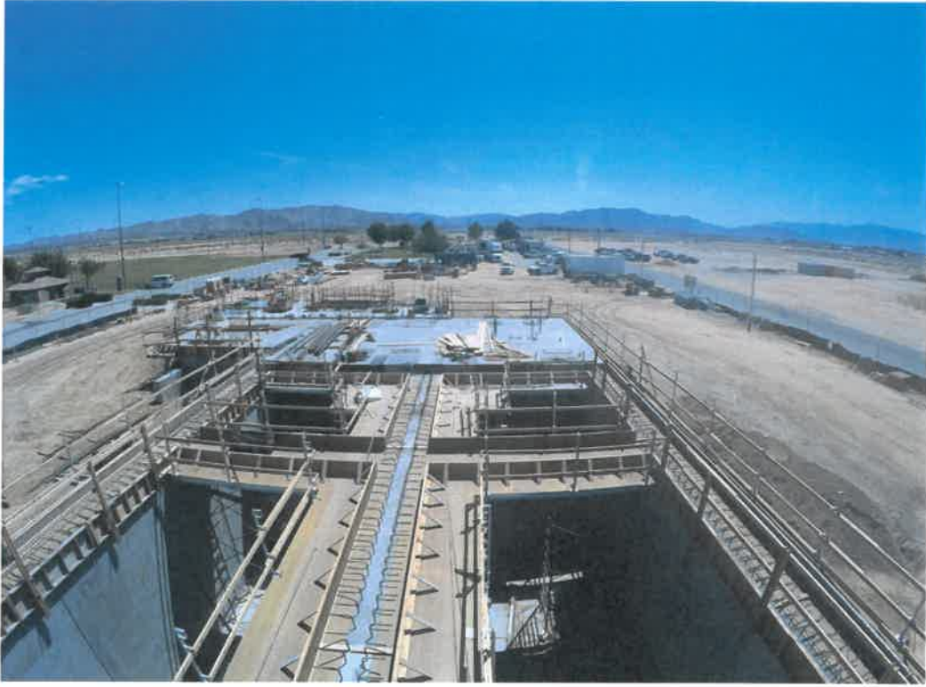
Apple Valley Sub-regional Water Reclamation Plant Project
