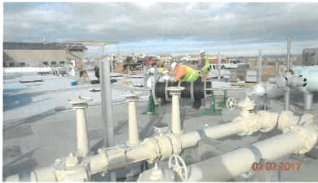
Hesperia Plant – under construction
