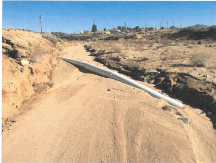
Figure 1.1 Exposed Interceptor
