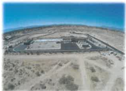
Hesperia Sub-regional Plant
