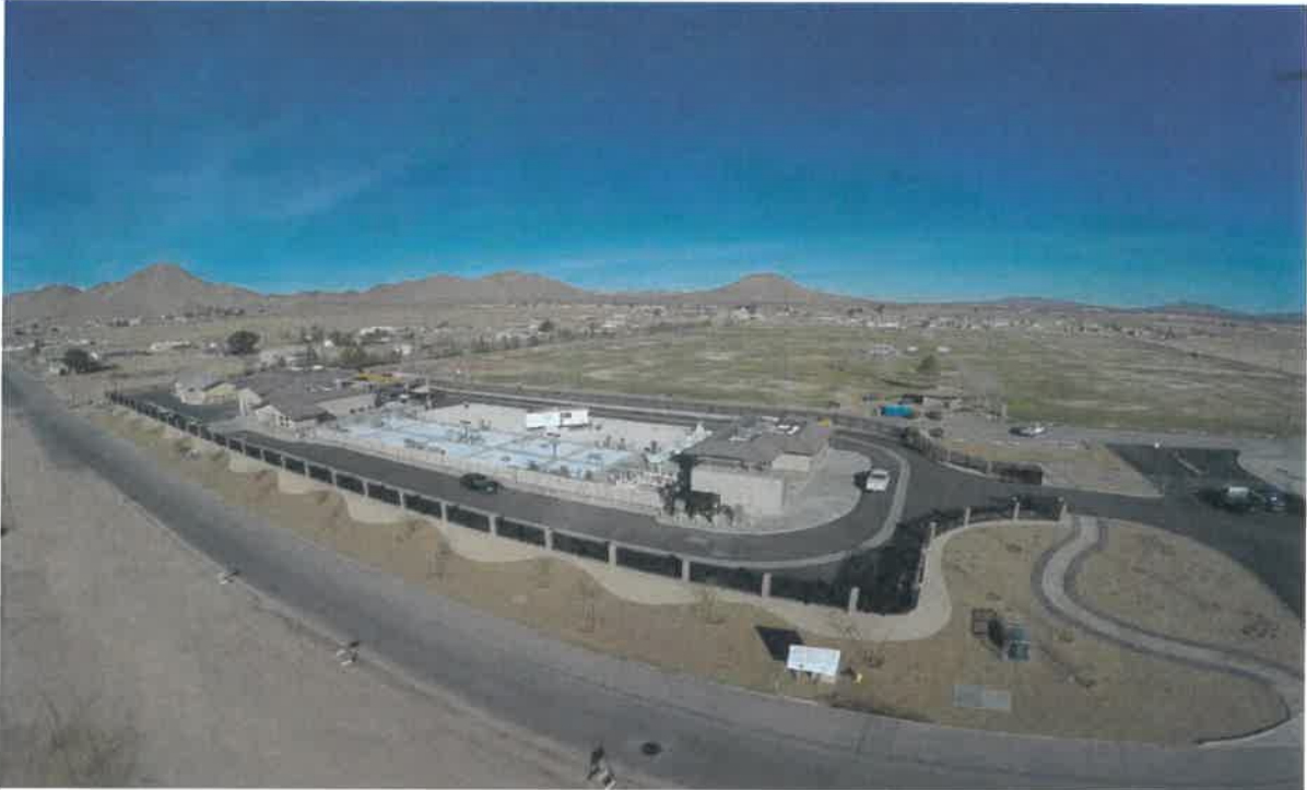
Apple Valley Sub-Regional Water Reclamation Plant
