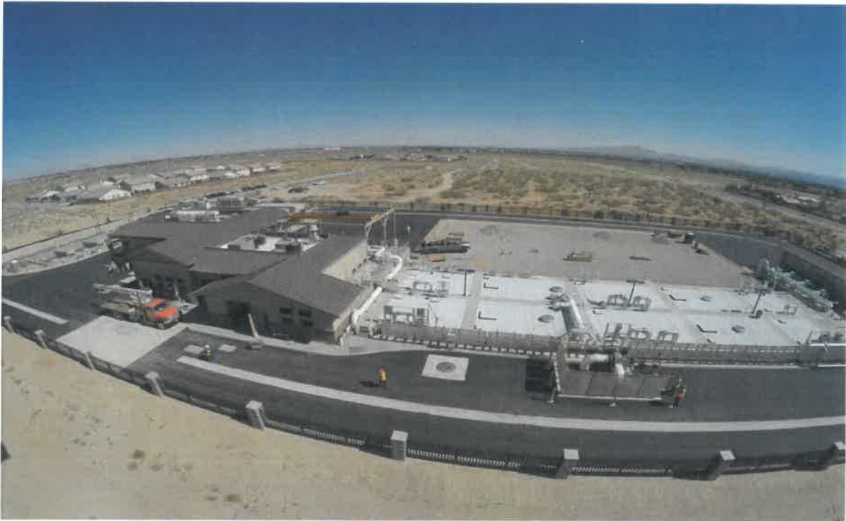
Hesperia Sub-Regional Water Reclamation Plant
