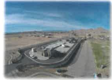
Apple Valley Sub-regional Plant
