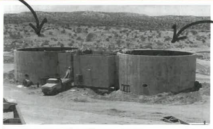
Construction of the original digesters in 1979.
