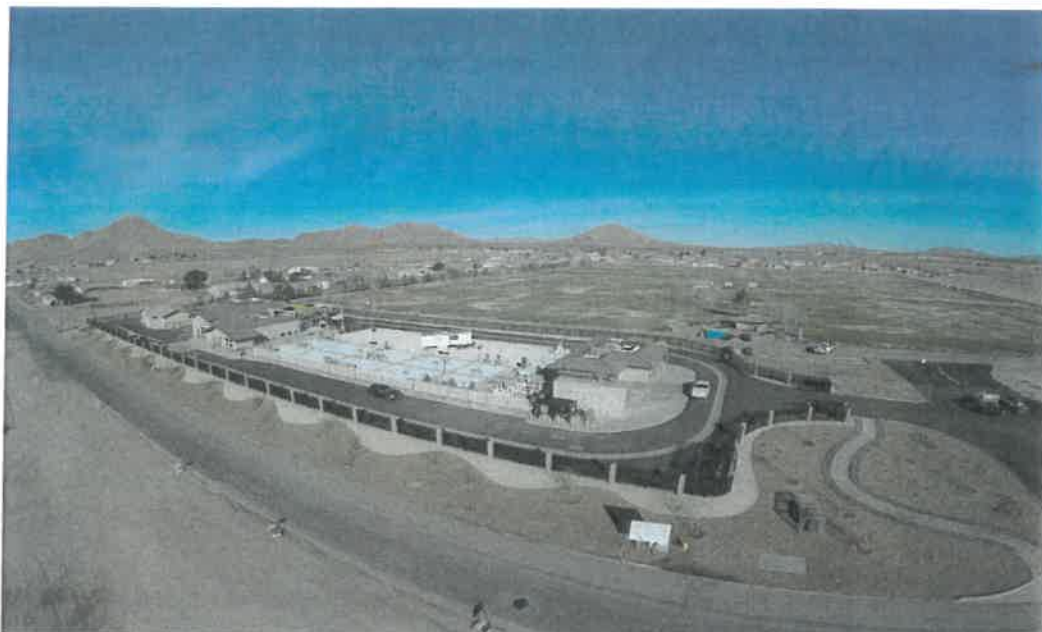
Apple Valley Sub-regional Water Reclamation Plant Project
