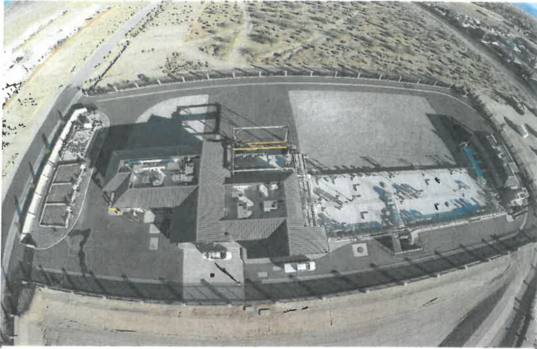
Hesperia Wastewater Reclamation Plant
