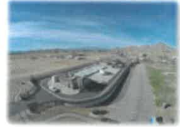
Apple Valley Sub-regional Plant
