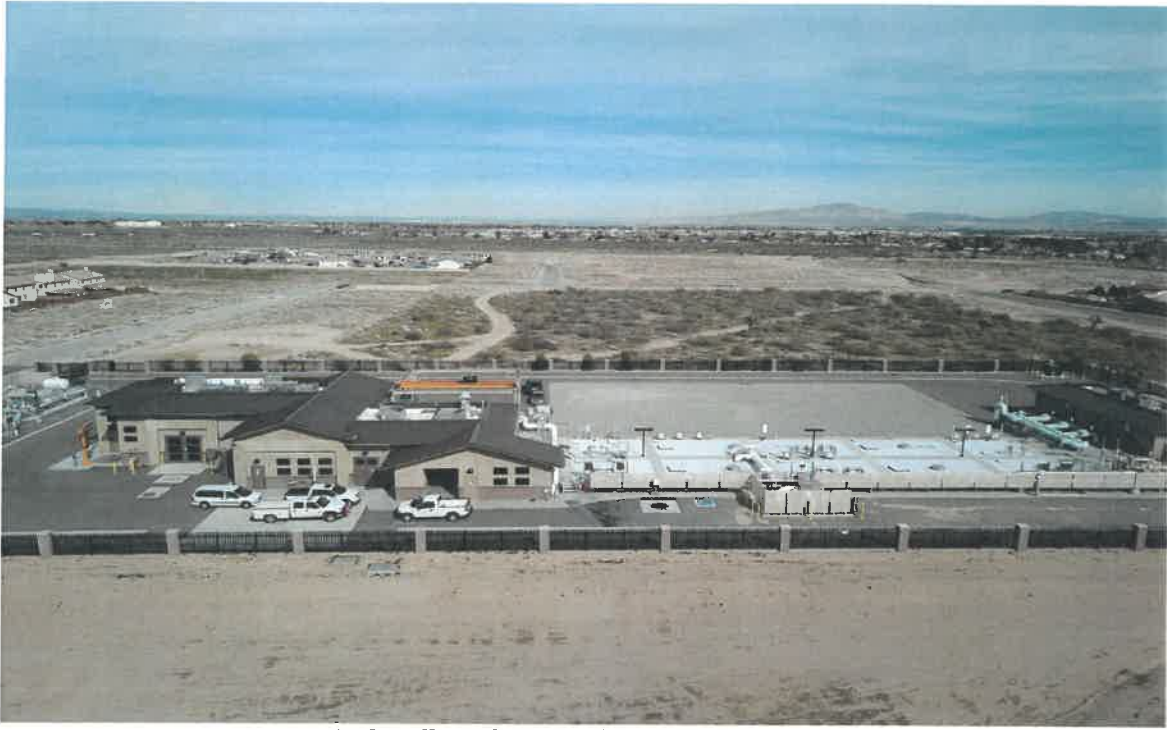
Apple Valley Sub-Regional Water Reclamation Plant
