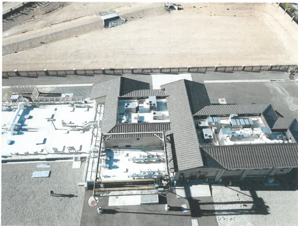
Hesperia Sub-Regional Water Reclamation Plant
