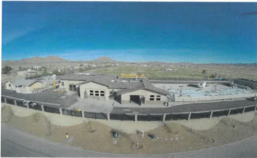
Apple Valley Wastewater Reclamation Plant
