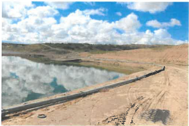
Percolation Pond at the Regional Plant
