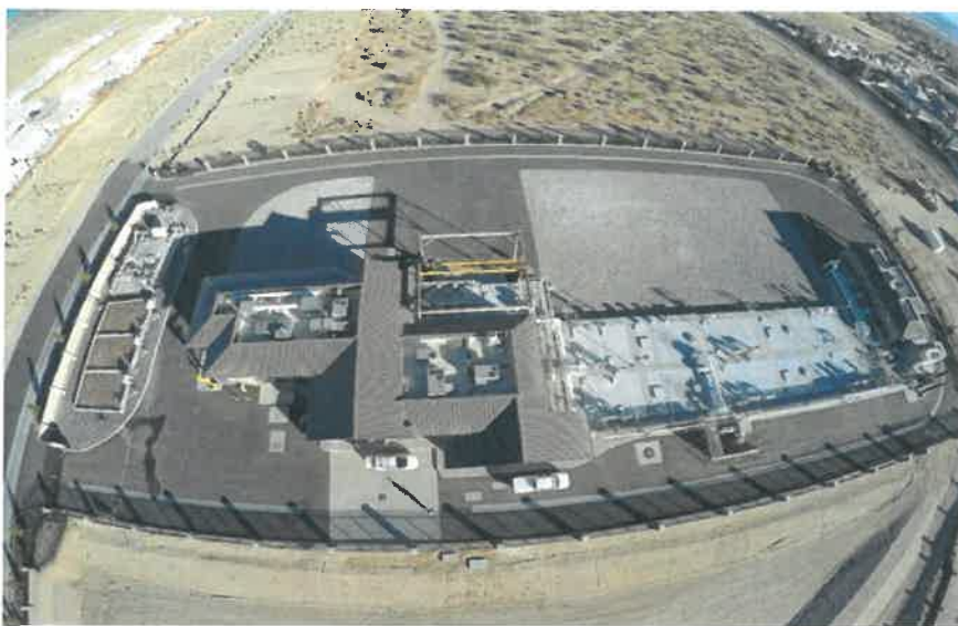
Hesperia Wastewater Reclamation Plant
