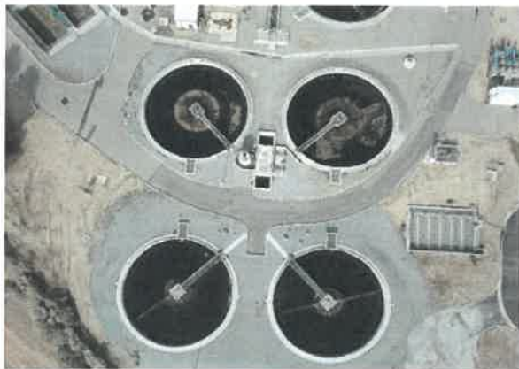
Regional Secondary Clarifiers
