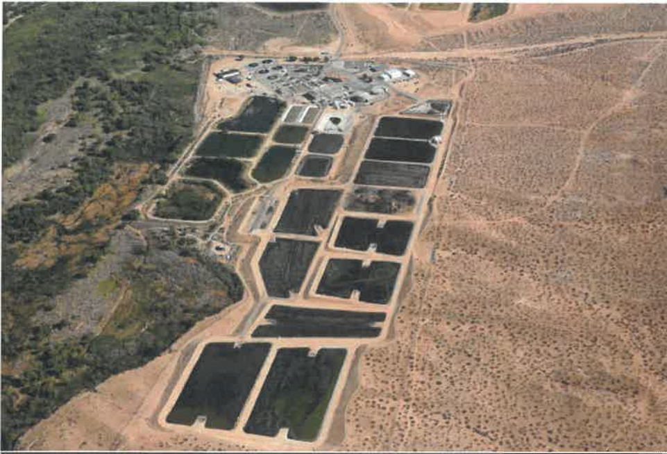
VWRA Regional Plant
