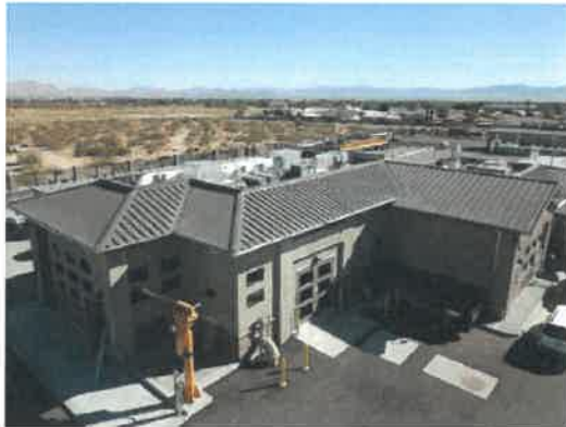
Hesperia Wastewater Reclamation Plant
