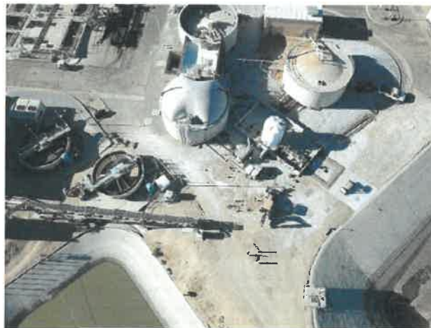
Regional Plant Digesters
