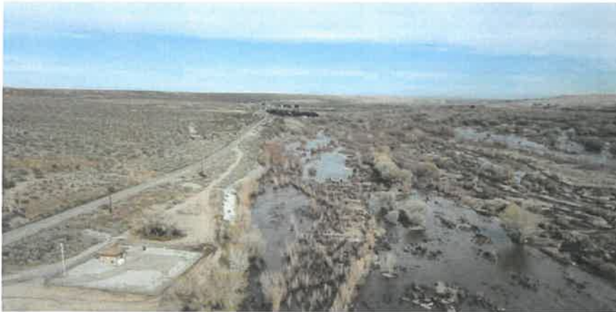
Oro Grande Pump Station
