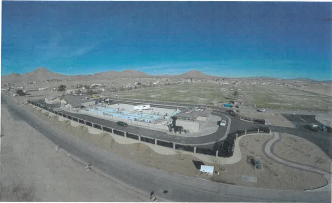
Apple Valley Sub-regional Water Reclamation Plant
