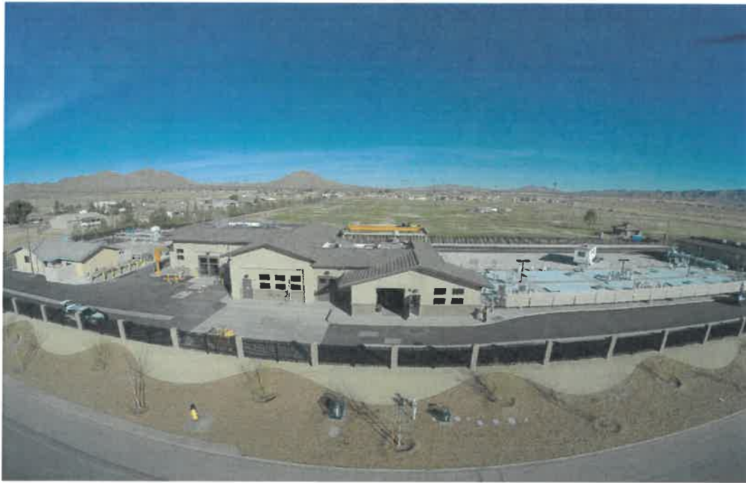
Apple Valley Wastewater Reclamation Plant
