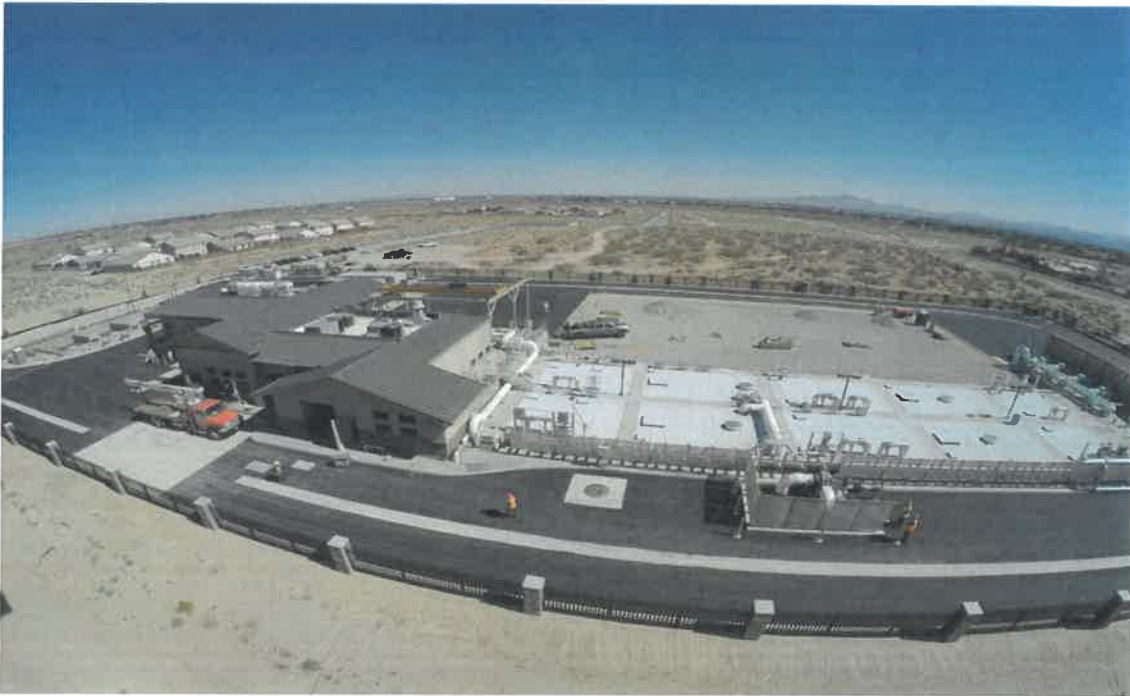
Hesperia Sub-regional Water Reclamation Plant
