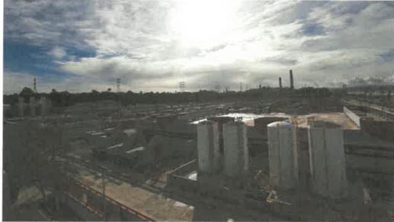
A view of the Hyperion Water Reclamation Plant in Los Angeles on Feb. 21, 2019. (Genaro Molina / Los Angeles Times)
